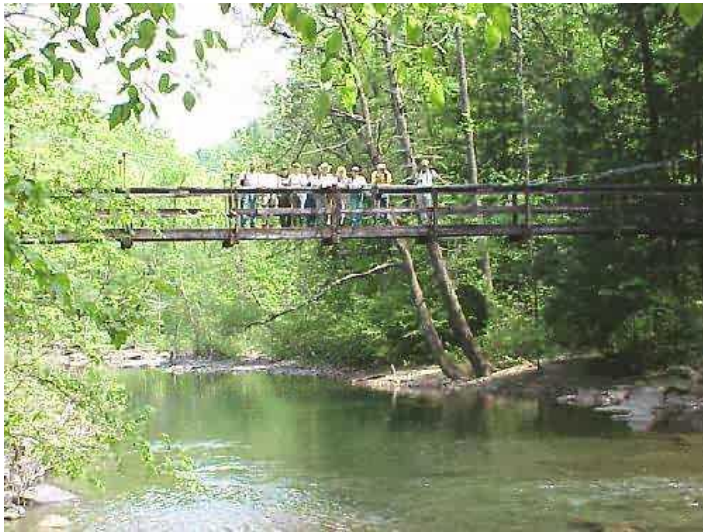
Bridge over Piney River
